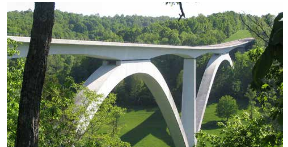
Natchez Trace Parkway Bridge
