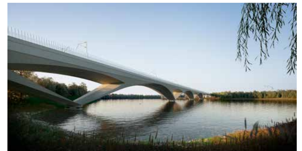
Colne Valley HS2 Viaduct
