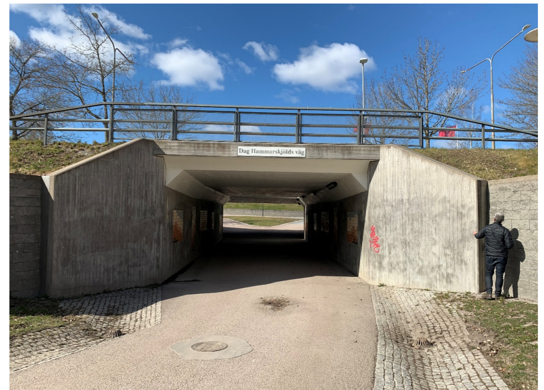
Befintlig situation. (Bild, Bjerking)
