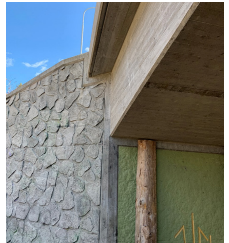
Befintlig situation. (Bild, Bjerking)
